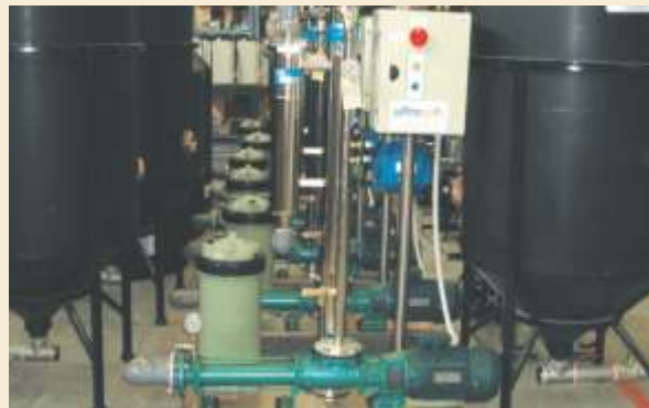
Battery of RD512 Pumps for Oil Water Separator application at Australia
