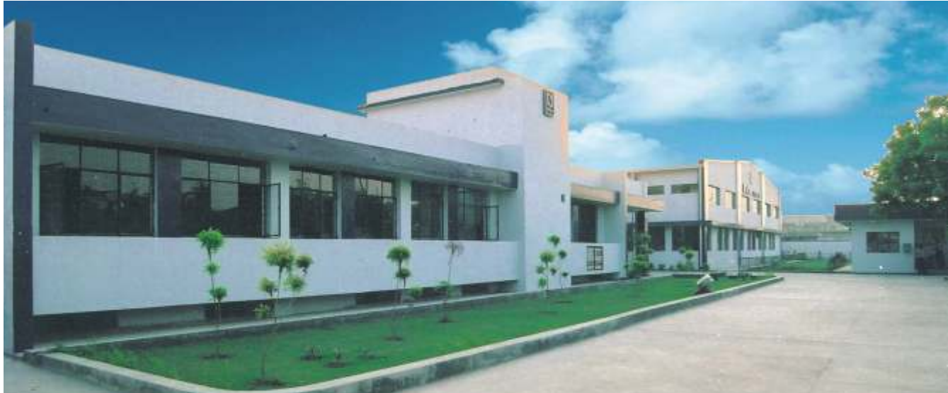
Roto's Manufacturing Plant
