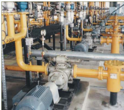
Twin Screw Pump pumping Lube Oil at Lube Oil Blending Plant in Haldia, India
